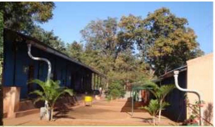
PHOTO # 6 : SHOWING RAIN WATER HARVESTING STRUCTURE FOR GROUND WATER RECHARGE @ CAMP AREA
