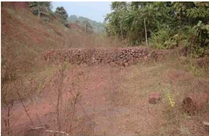
PHOTO # 4B: SHOWING CHECK WEIRS & SETTLING PIT PROVISIONS AT THE STRAGIC LOCATIONS TOWARDS PREVENTIONS OF THE MINES SURFACE RUN OFF BEFORE FINAL DISPOSAL TO OUTSIDE WATER BODIES
