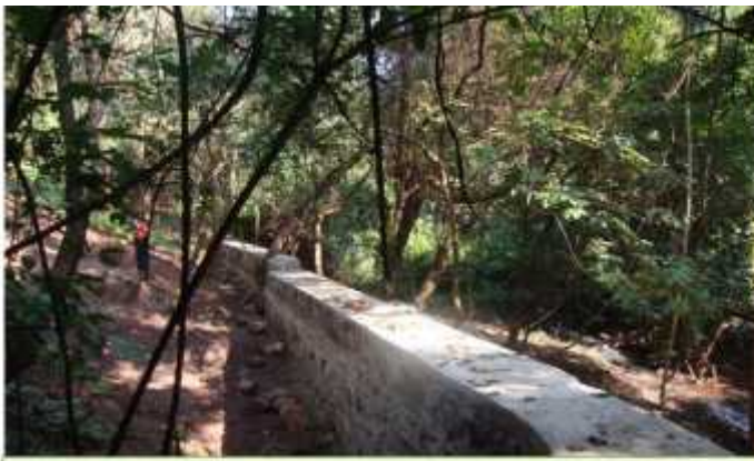
PHOTO # 5 : SHOWING GUARD WALL ALL ALONG THE NALLAH
